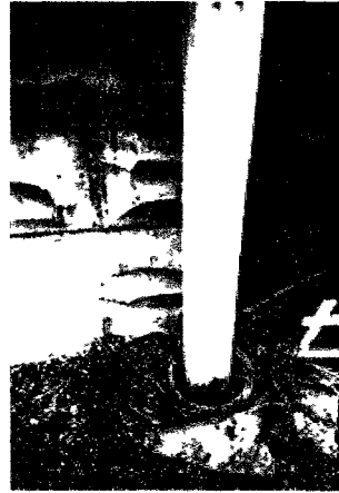
Figure 2.2 Example of Inflow: A Down Spout Connected
