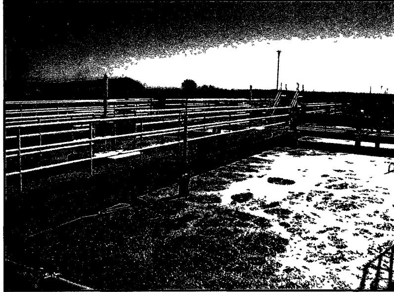
Figure 4.2 Fine Bubble Diffusers Used to Aerate Wastewater
