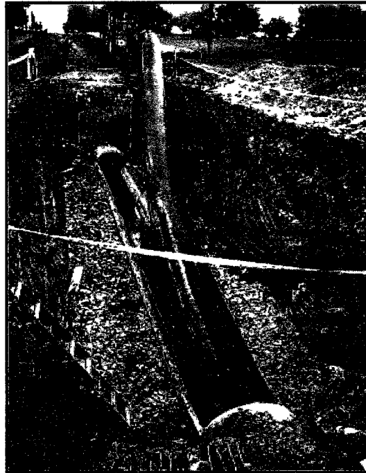
Figure 9.6 Pipe Bursting in Progress
